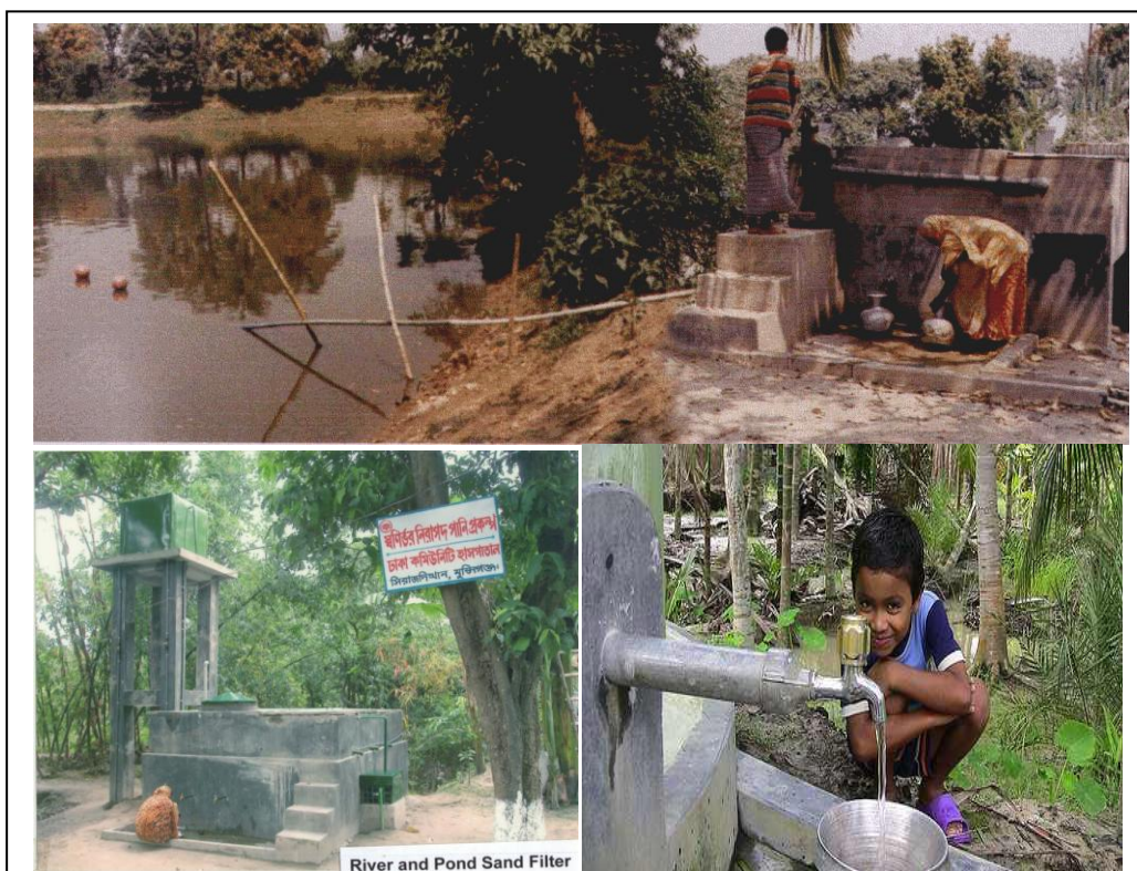
Figure 5 Pictures of Pond Sand Filter
