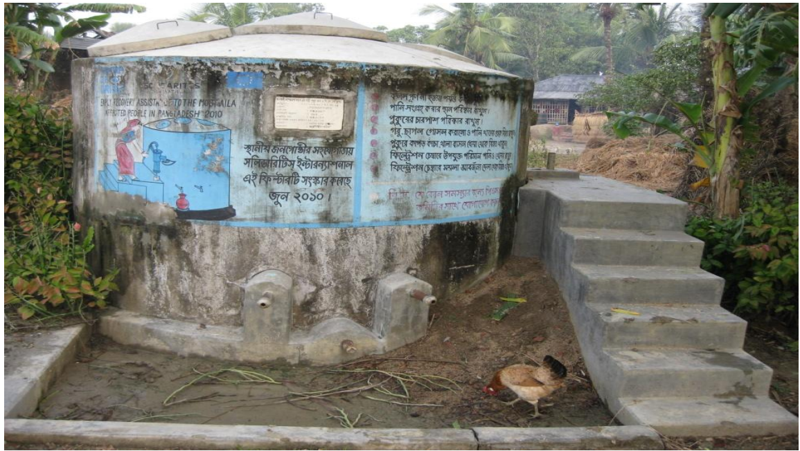
Figure 9 A non-functional PSF in Dhankhali and abandoned pond below which had been inundated with saline water during Aila
