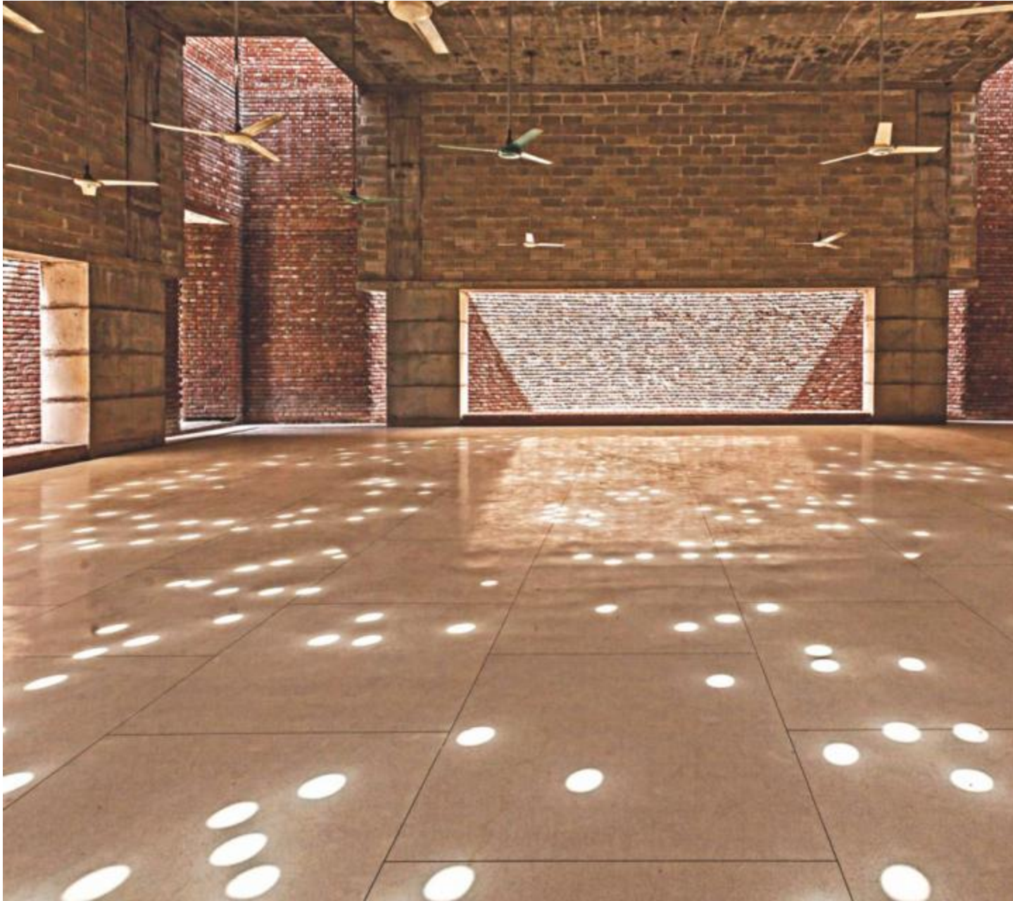
In addition to four light courts, random circular roof openings allow daylight into the prayer hall creating an ornate pattern on the floor enhancing spirituality through light. Bait Ur Rouf Mosque, Dhaka, Bangladesh, designed by Marina Tabassum. Photo: AKTC/Hassan Saifuddin Chandan
