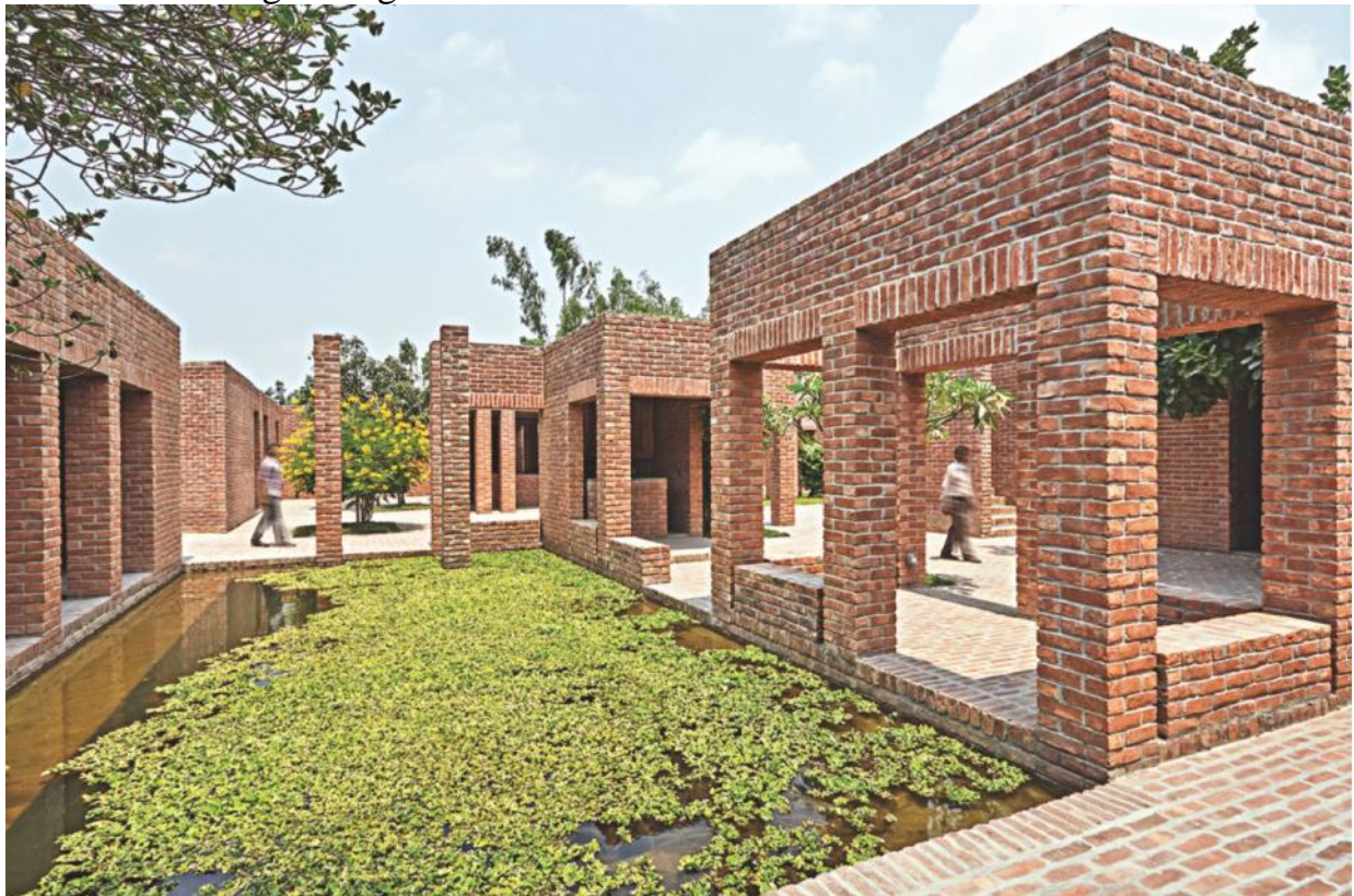
Located in rural Gaibandha where agriculture is predominant, the project's roofscape merges with its environment. Friendship Centre, Gaibandha, Bangladesh, designed by Kashef Mahboob Chowdhury. Photo: AKTC/Anup Basak
