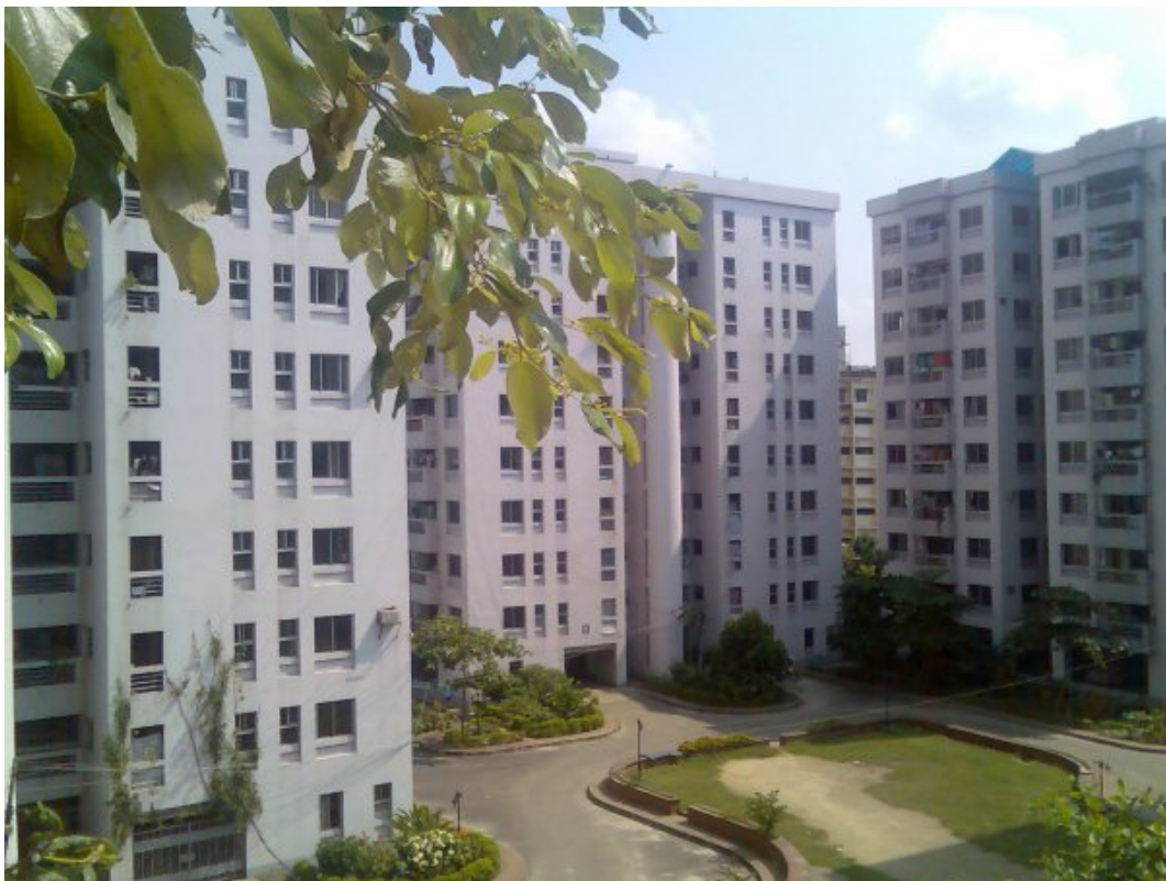
Figure 2.5.3: NAM Village, Housing Complex for Government Officers. Source ( http://www.panoramio.com/photo/20230989 )
