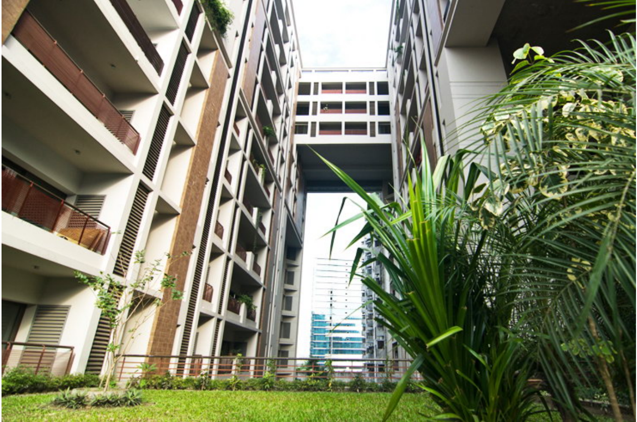
Figure 4.1.5: Spaces inside the building.
