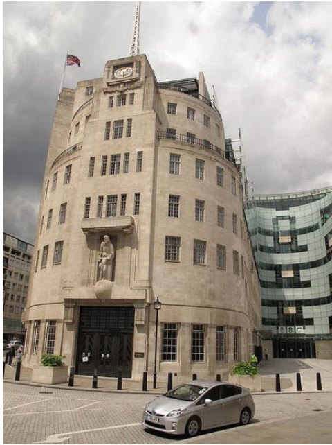
Figure 5.3.1 BBC Broadcasting House (Source: Google)
