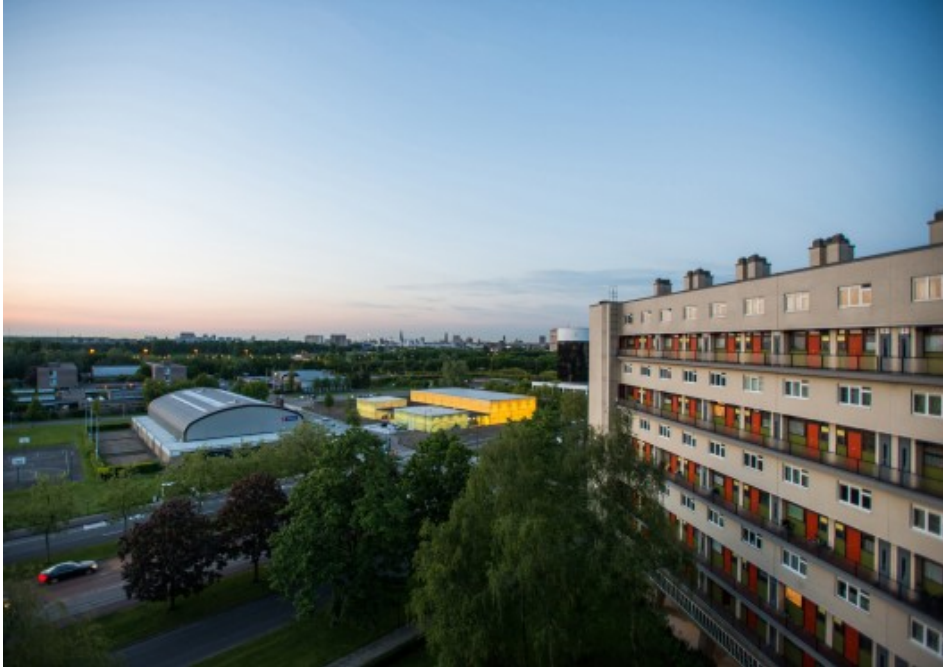
Fig 27: Photograph of Neighbourhood Sports Centre Kiel
