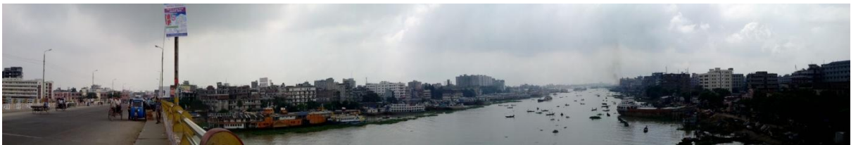
fig: View from top of the bridge
