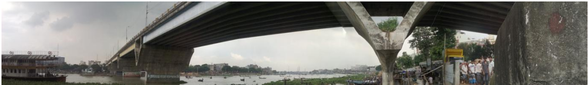
fig: Babubazar Bridge connecting old Dhaka with Keraniganj
