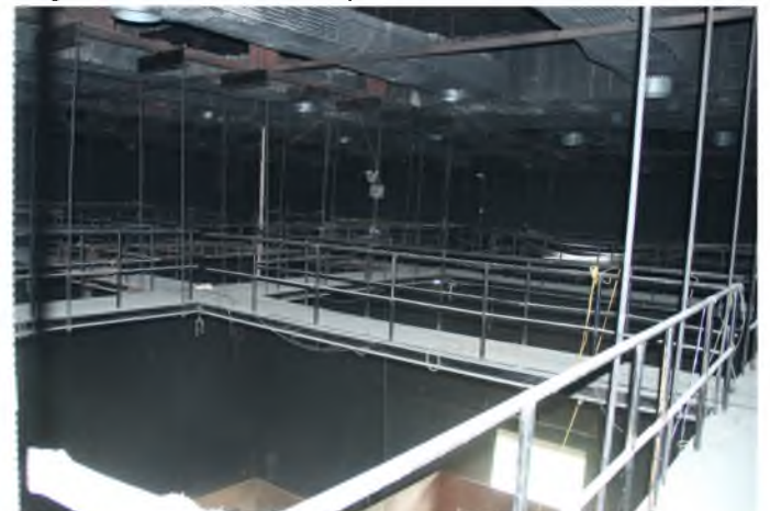
Fig 35 : Catwalk of the studio stage
