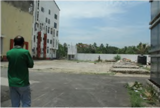
Fig 28 : Entry of the studio complex
