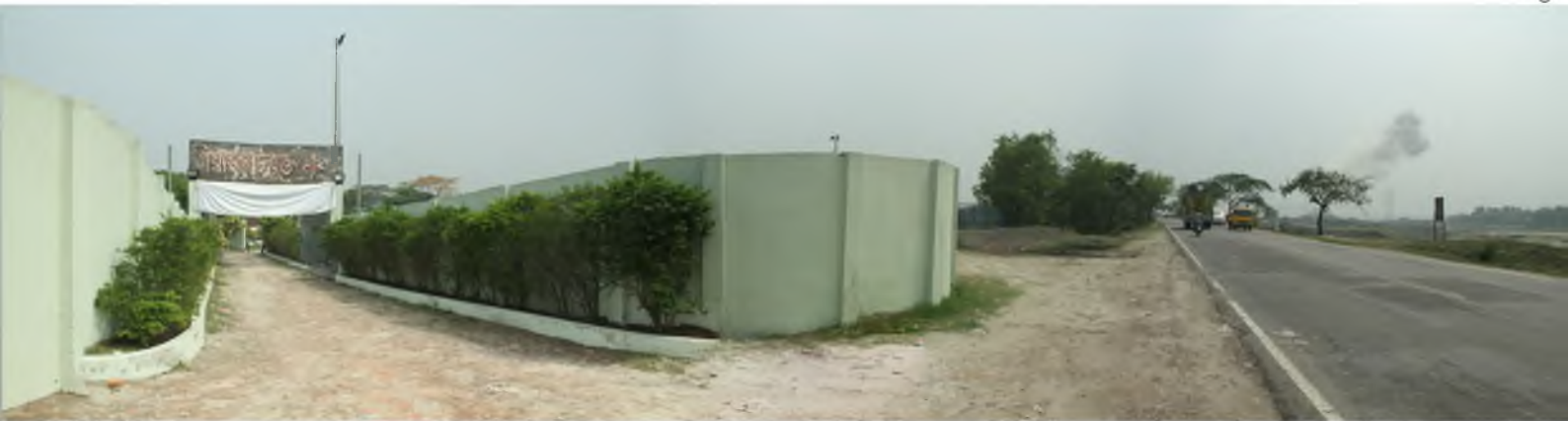
Fig 08 : Entry slope from the roadway
