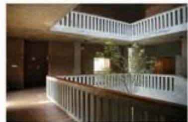
VIEW OF CIRCULATION AREA AROUND ATRIUM
