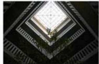
VIEW OF SKYLIGHT ABOVE ATRIUM
