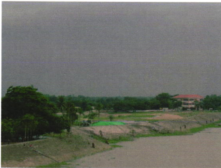
Figure 16: Photos of the site access road showing current condition (Rahman, 2013)
