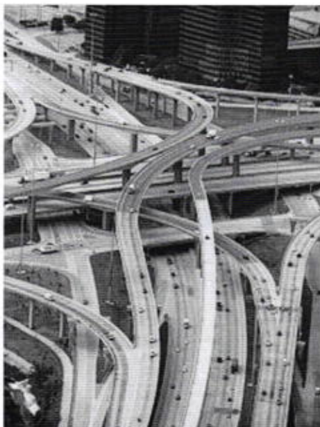
Figure 1 High Five Interchange five level stack interchange with multiple overpasses in Dallas, Texas.
