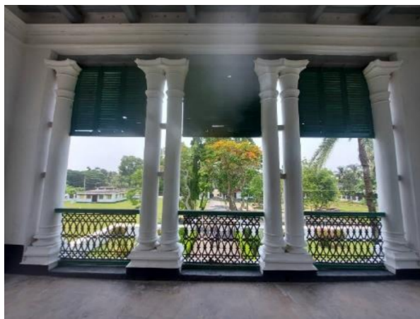
Figure: Inside the existing building
