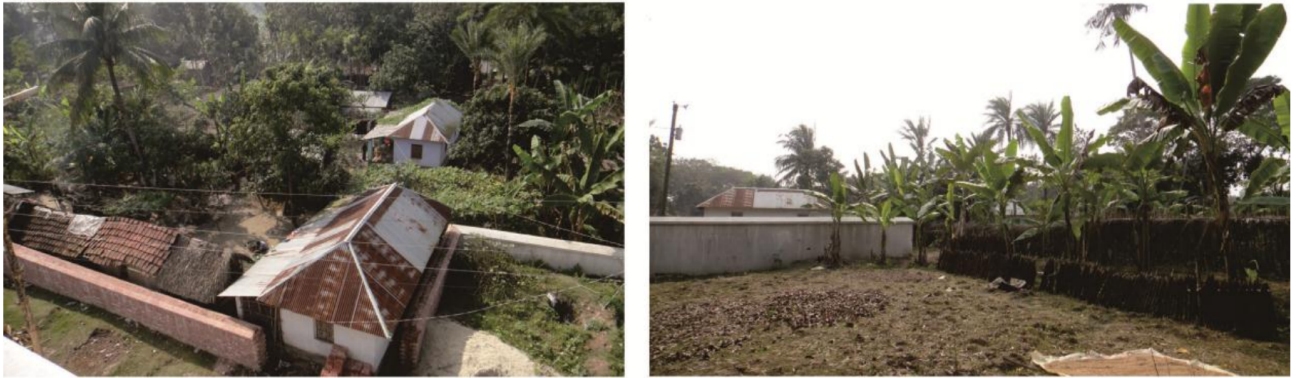
Figure: Low height tin shed residential houses
