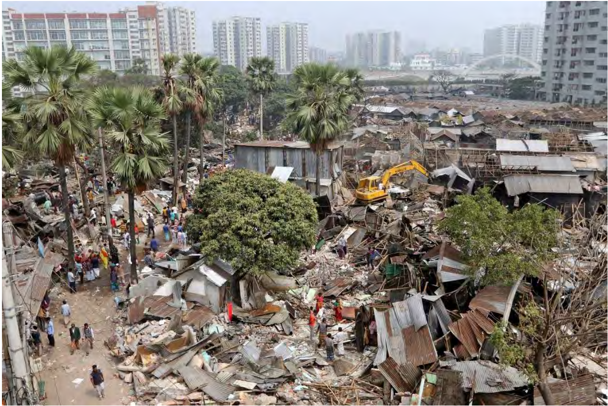
Figure 4.3.1: Image of demolishing the Bhashantek slum. Source: Google
