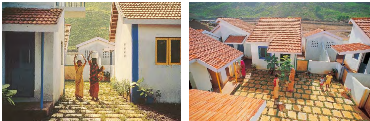
Figure 4.1.2: First image shows the human scale design increases community interaction. The second image shows a cluster, showing individual houses with the sanitary facilities along the same walls. Source: Google
