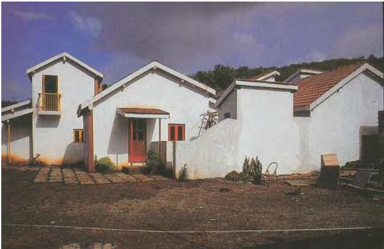
Figure 4.1.1: Belapur Incremental Housing, New Mumbai, India. Source: Google
