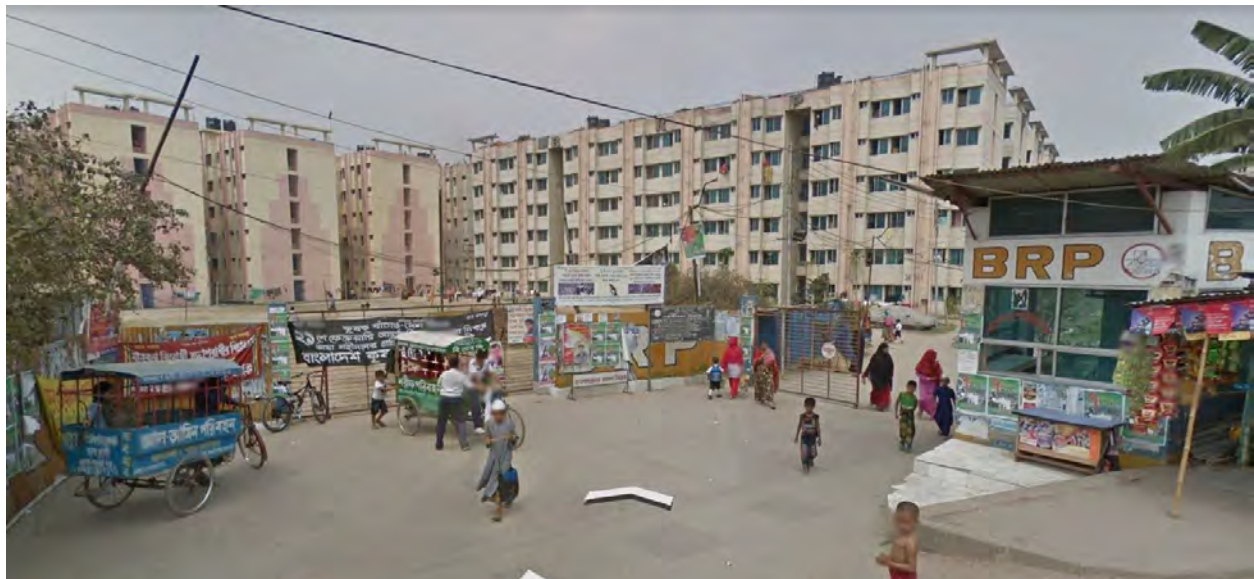
Figure 4.3.8: Image showing the existing condition of BRP. Source: Google Earth
