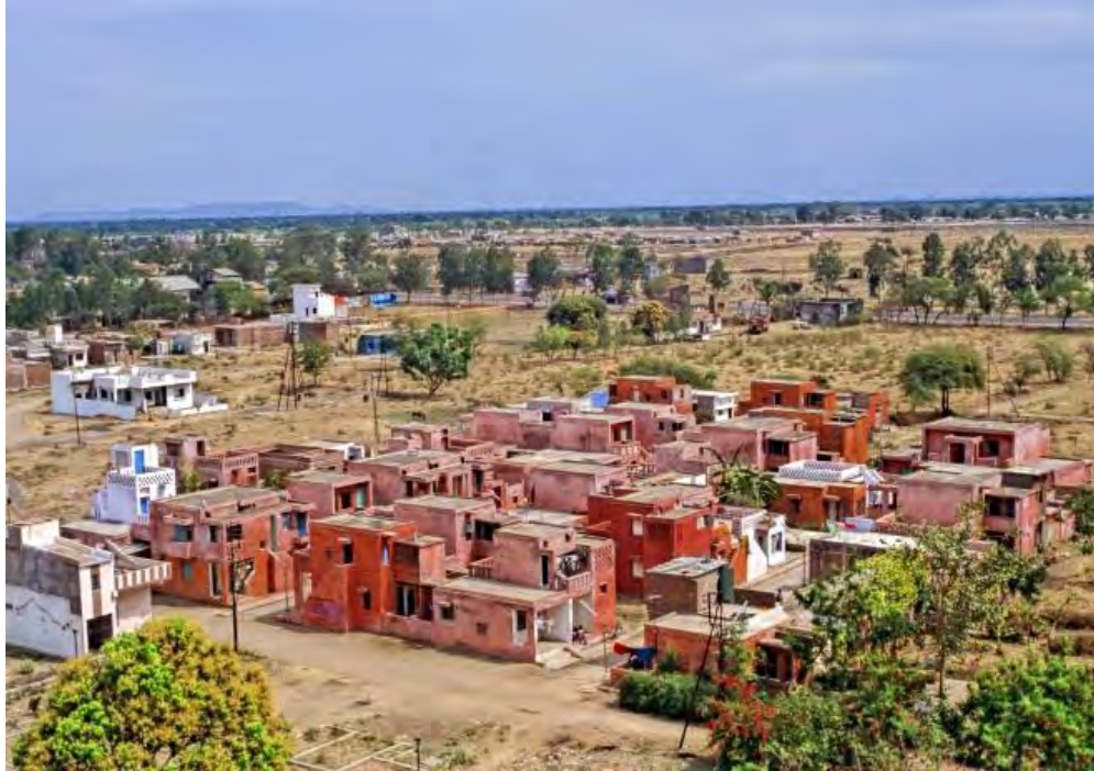
Figure 4.2.6: Images of Aranya Community Housing. Source:Google
