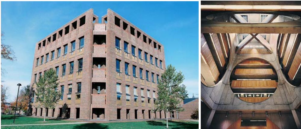
fig 24: Outer walls taper towards top (left), Central cross-beam support (right). Source: Archdaily
