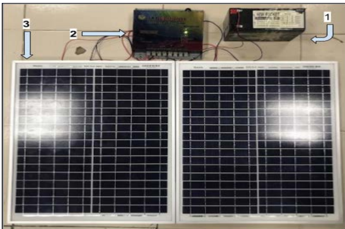
Figure 29: Solar Panel Installation (1.12V battery, 2. Solar charge controller, 3.20W solar cell).
