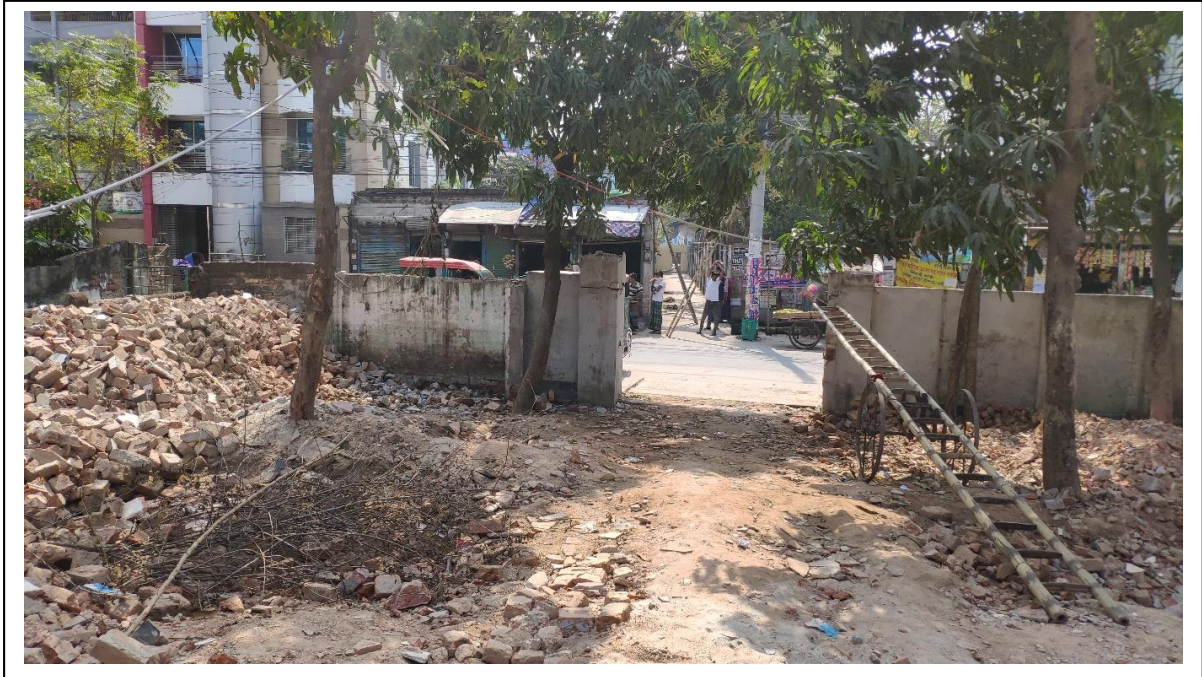
Image 3: view towards the main access road from site (Source: author)
