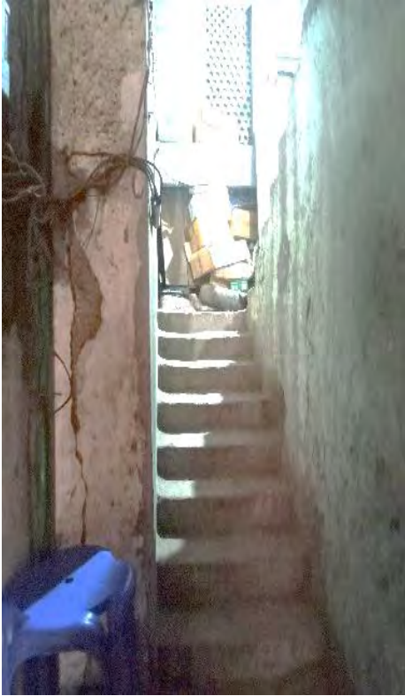
Figure 40: staircase of Sample 2.
