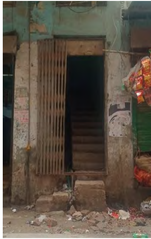
Figure 41: staircase of Sample 3.
