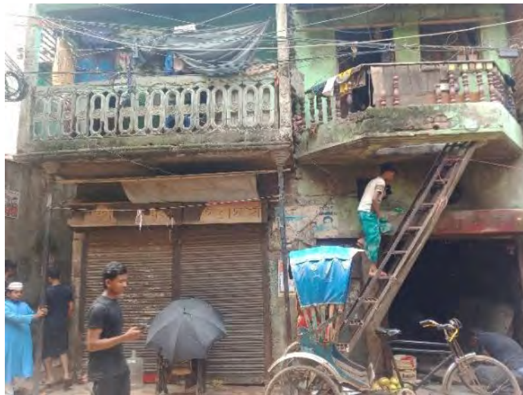
Figure 42: staircase of Sample 4.
