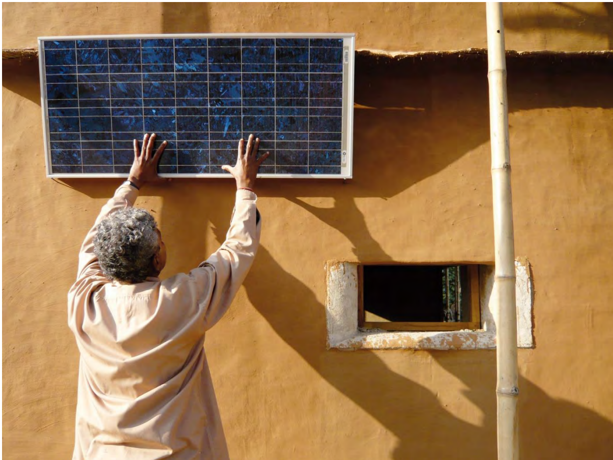
Figure 4.3.4: Installation of solar panel
