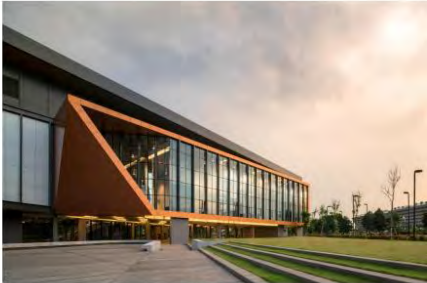
Fig 4.1.2: CAT Telecom Headquarters
