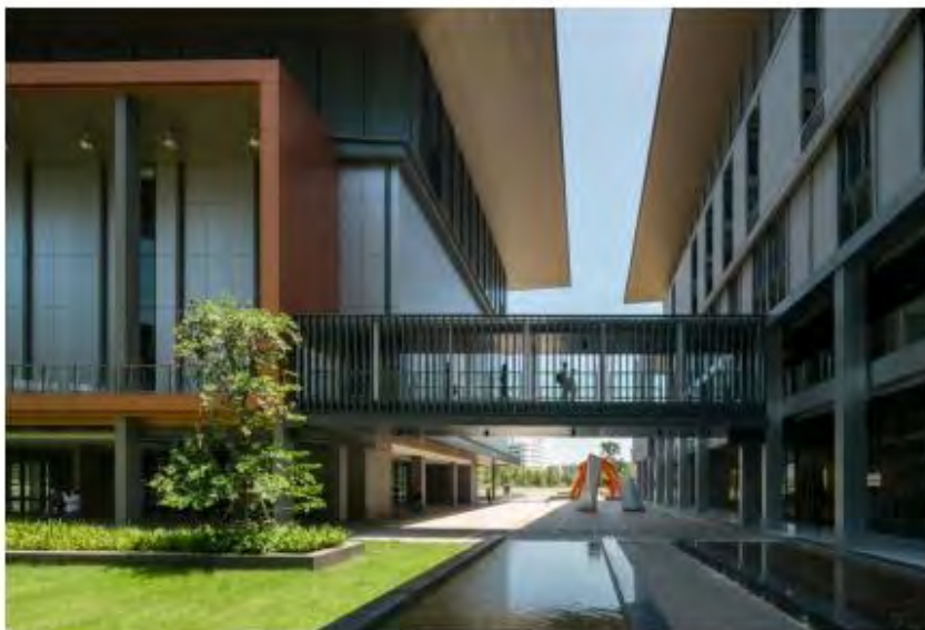
Fig 4.1.3: CAT Telecom Headquarters
