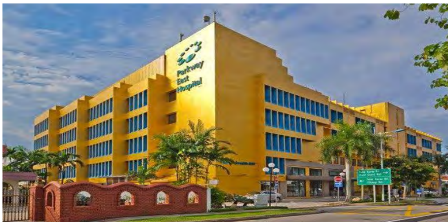
Figure (6): Parkway East Hospitals
