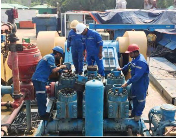
Maintenance of Rig Pump
