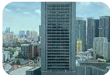
Singtel Telecom Tower Singapore
