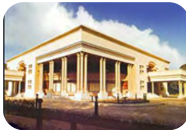
VVIP Rest House
