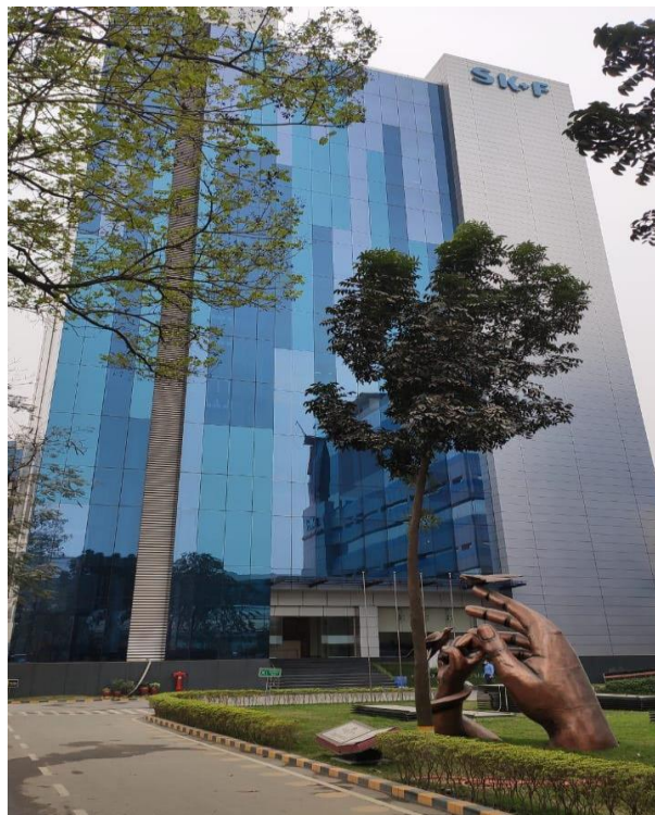
Figure 1: Tongi Manufacturing Facility, Eskayef Pharmaceuticals Limited
