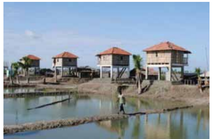
Our students designed and built 43 houses in Satkhira as Disaster Resilient Habitat for the families affected in the flood-prone area
