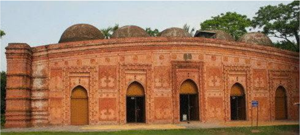
Figure 2.3.3.b: Pathrail Mosque, Faridpur
