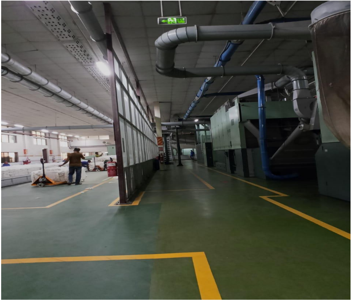
Fig no-04: Blowroom (Photo by Atiqur in July 30,2022)
