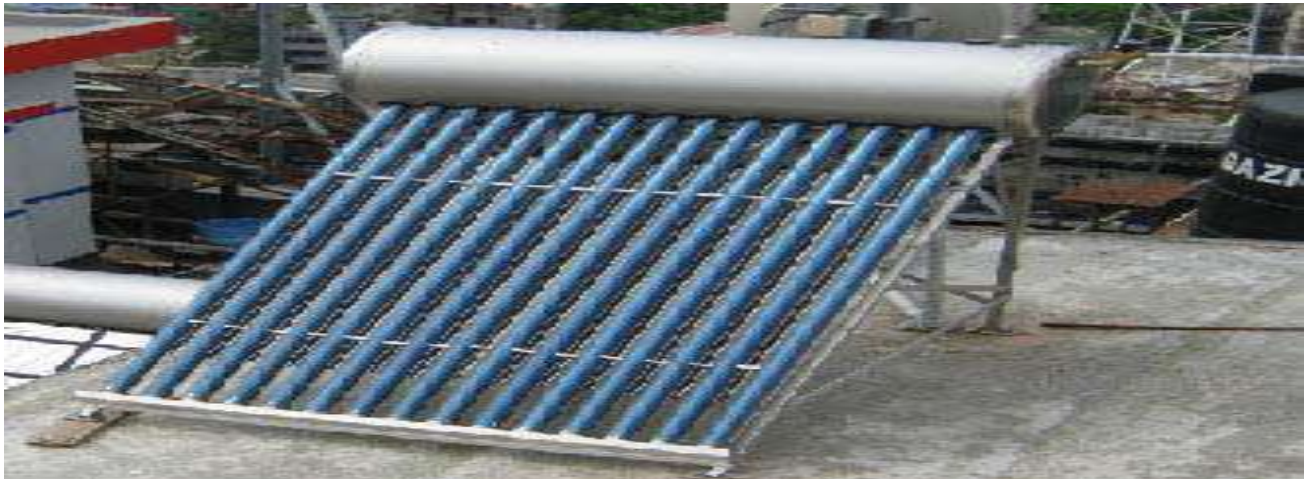
Fig.5: 150 liters tank with directly connected water-in-glass evacuated tube collectors
