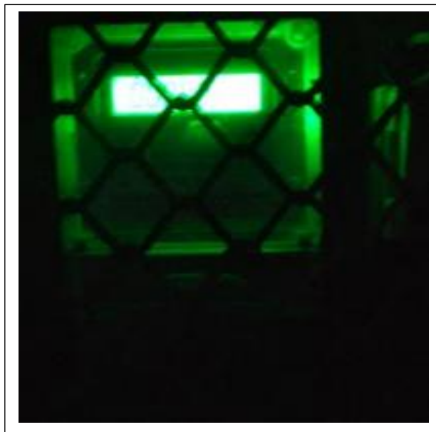
Figure 2.32: Meter from 2 nd apartment of Faridabad (night view)
