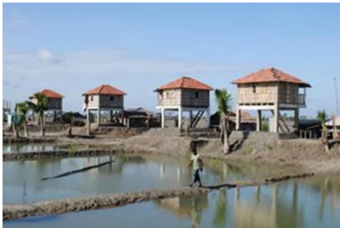
Our students designed and built 43 houses in Sathkira as Disaster Resilient Habitat for the families affected in the flood-prone area
