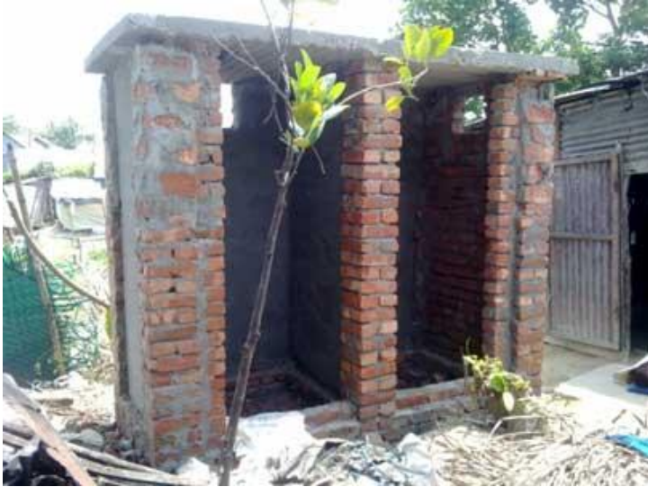
An interventions in one of the treatment slums: building sanitary latrines
