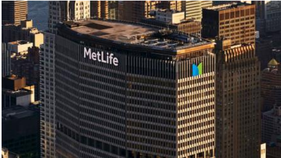
Figure 5 MetLife Headquarters at NY, USA
