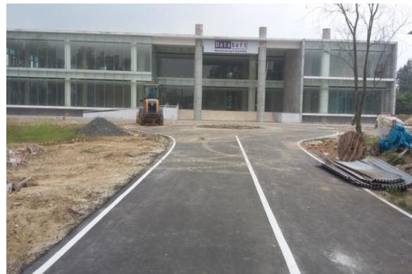
Constructed Service Building
