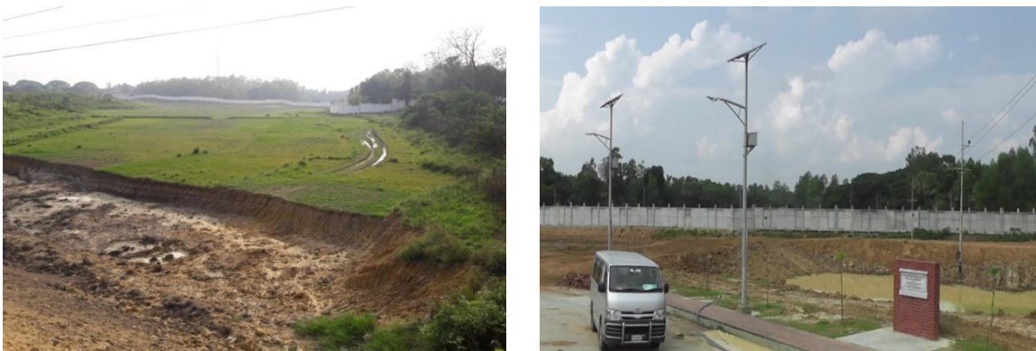
Newly constructed boundary wall
