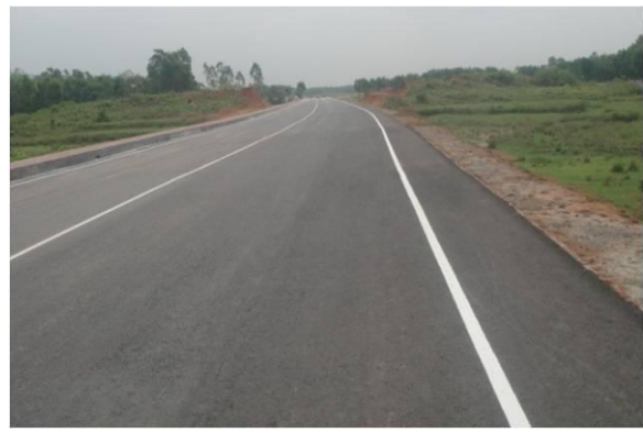
Internal Access Road
