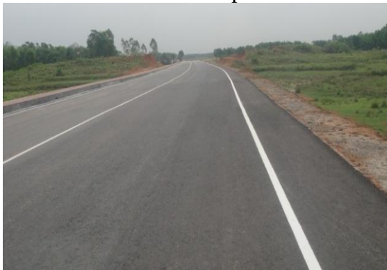
Internal Access road of Bangabandhu Hi-Tech City
