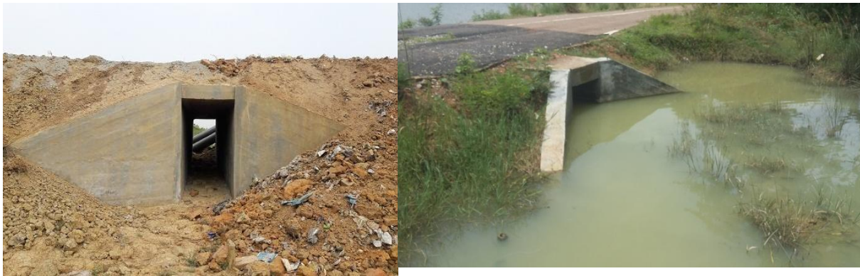
Culvert in BHTC
