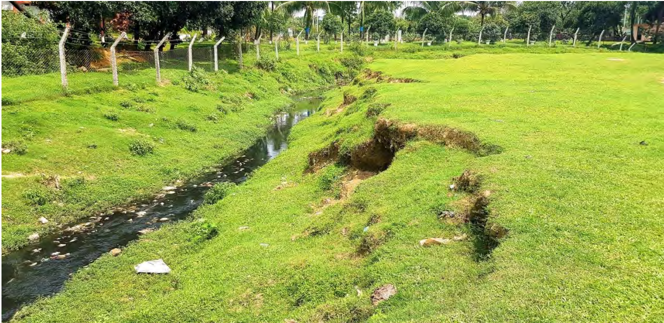
Canal by the west side of the site
