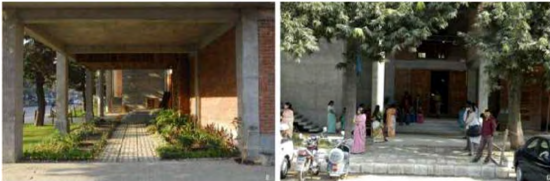
Fig39 :Exterior corridor and entrance
