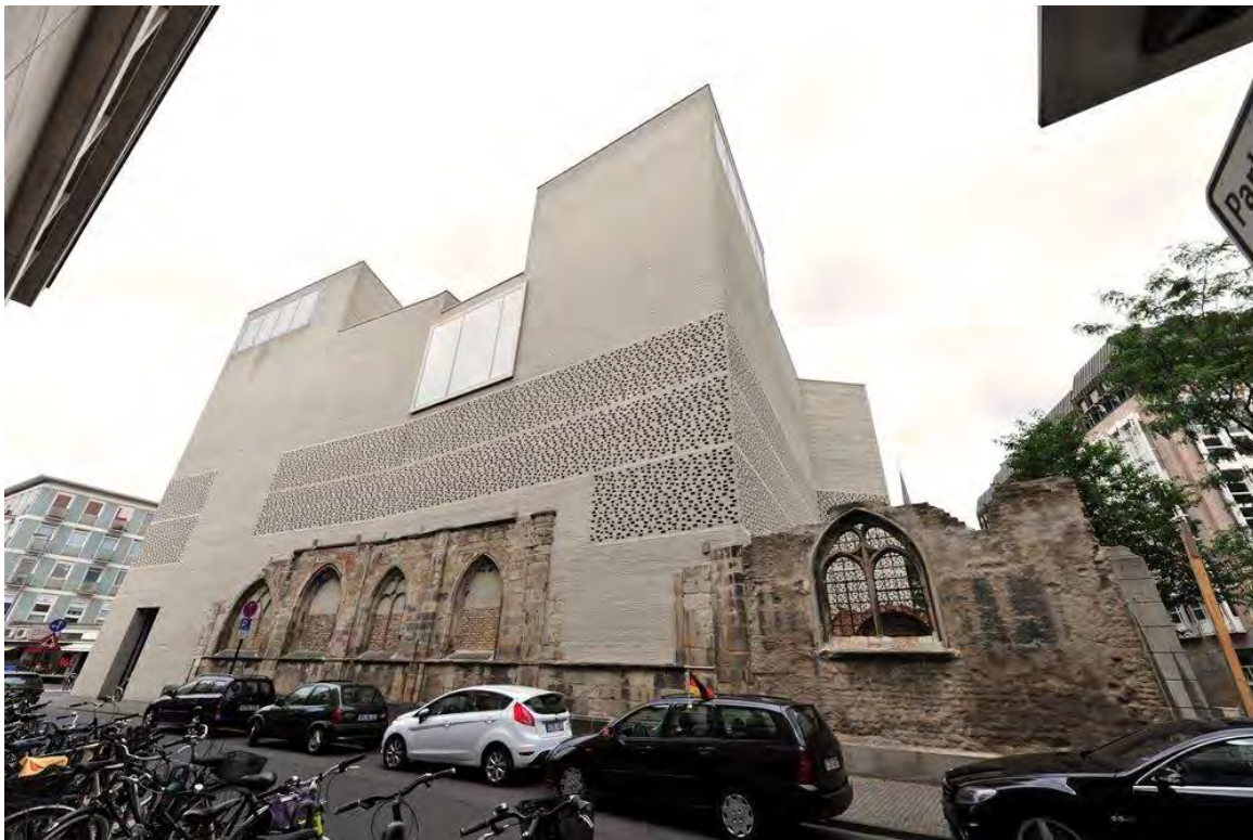
Figure: Street view, Kolumba Museum (Source: Archdaily)
