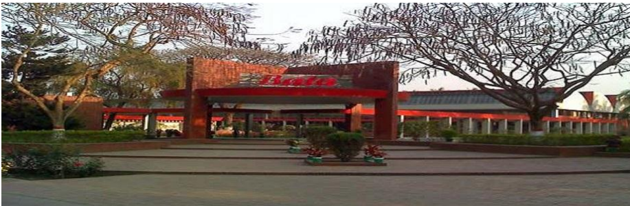
Pic: Dhamrai Factory
