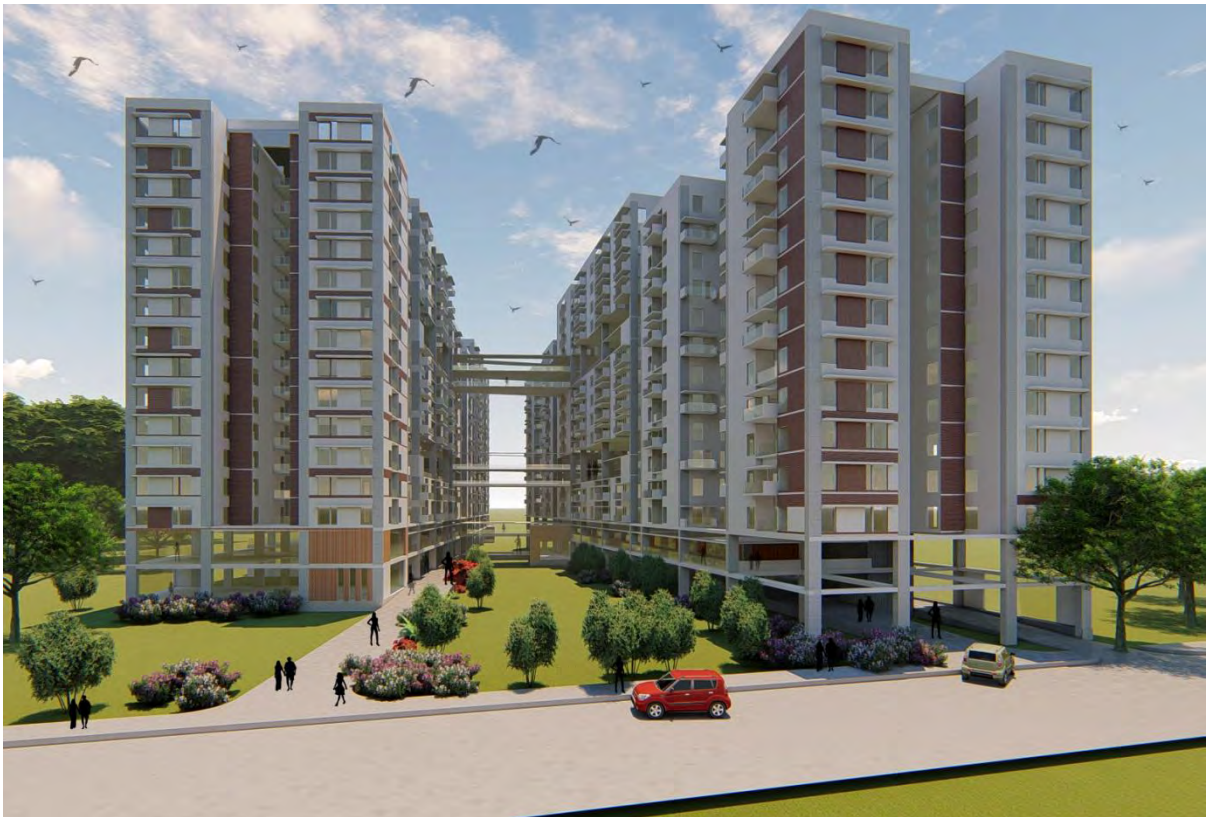
Figure 6.7.1 : View from the west (Source: Author)
