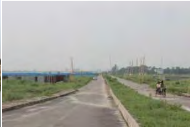
Figure 2.7: road at the front side
