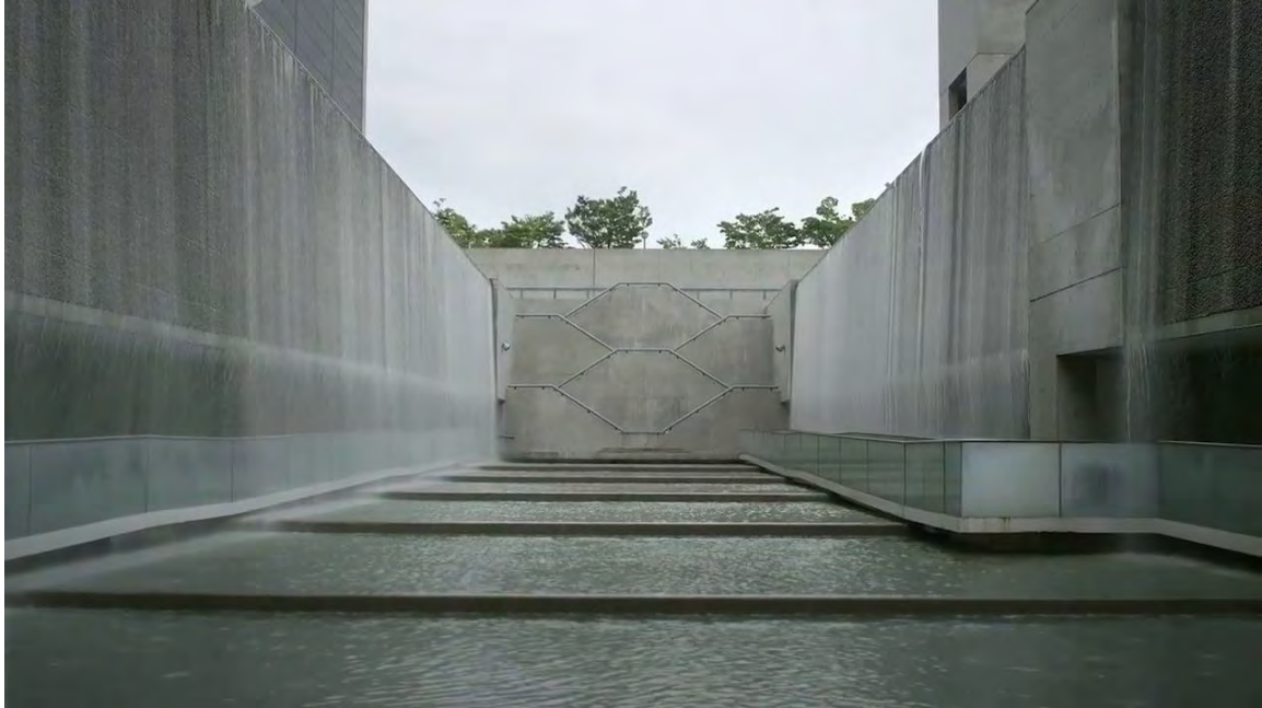
Figure: Water Curtain Side View Source: https://arcspace.com
