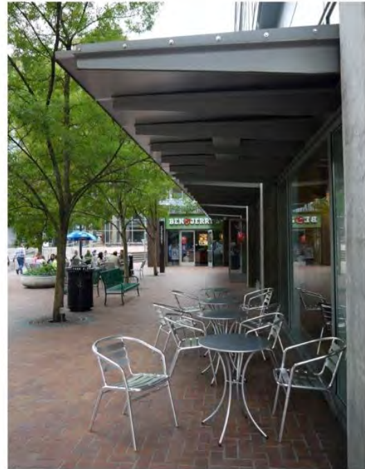
View from the northwest of lower plaza and cafe seating near restaurants
