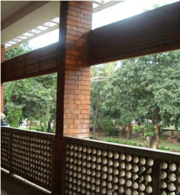
fig:051 shedding device and railing , source:
