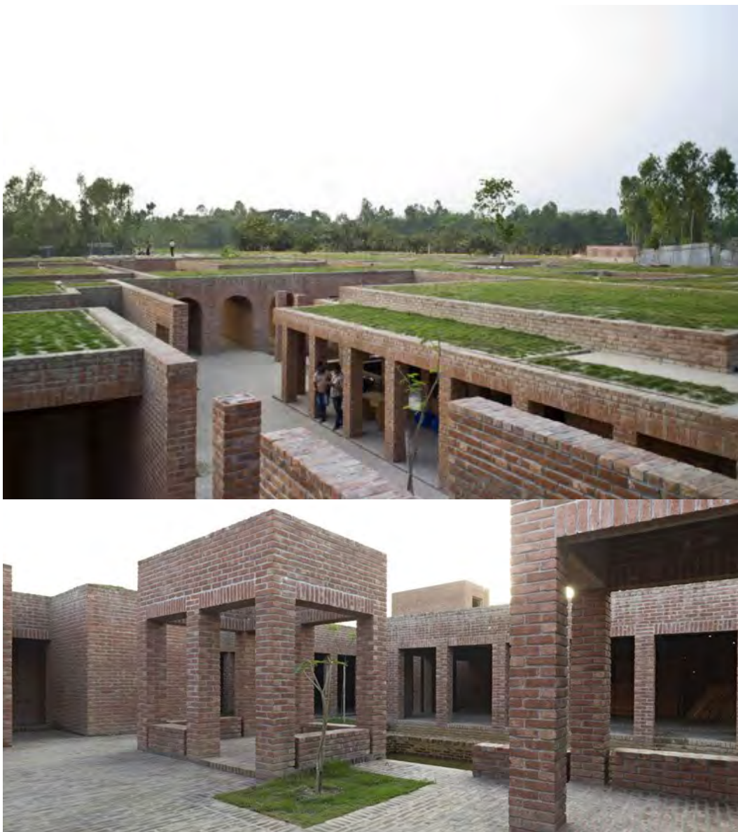
Fig 5.1.1 : outdoor spaces [Source : Arch Daily]
