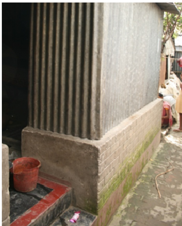
FIGURE 6 A house with half-brick wall (Type 4).
