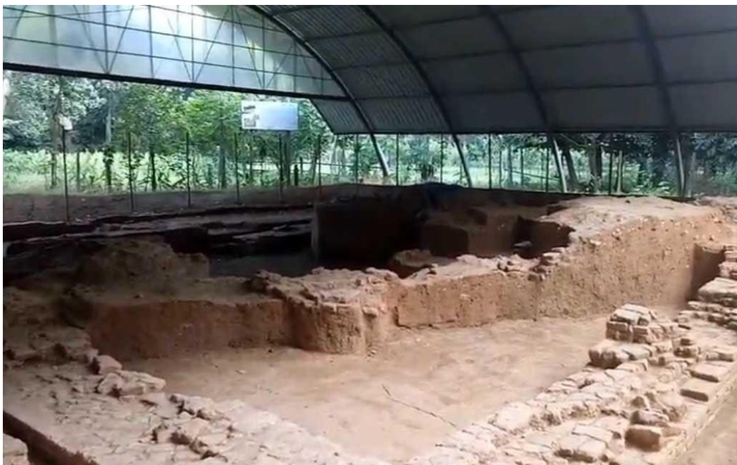
Figure 1: Tin and bamboo made canopied structure to protect the ruins and also visible for then visitors
