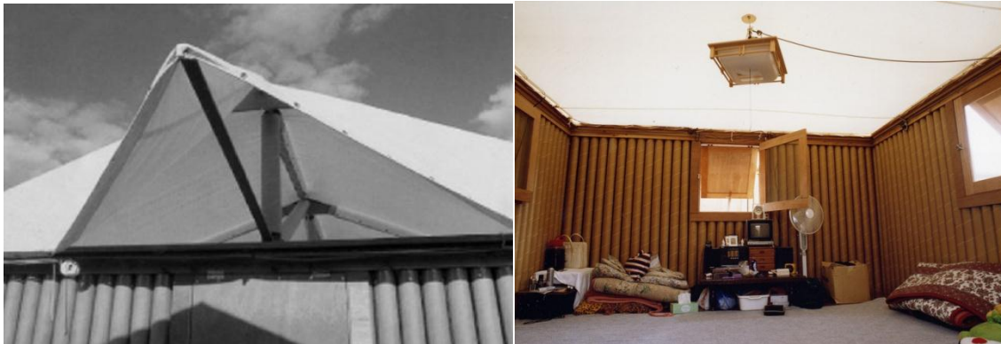
Figure 13. The hatch in the roof allows for air circulation and illumination of the interior (Source: http://www.houzz.com/ ; HBRC Journal(2014))
