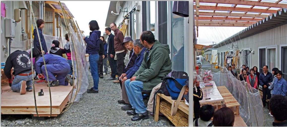
Figure 12 Installation of the poly-carbonate roof, wooden deck & frame and seating ( Source: MIT 3:11 report )
