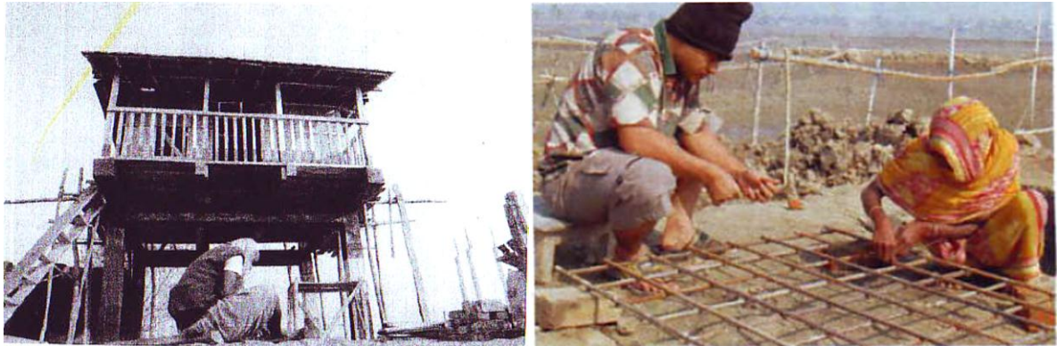
Figure 29. The test house being built in collaboration with the locals, students & architects (Source: Springer, CCA)
