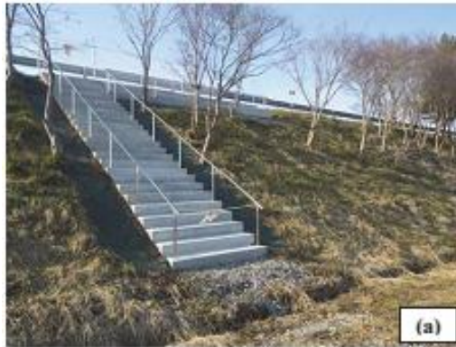
Figure 55 Concrete stairways being built for access to the surface of the expressway (Source: Journal NDS, 2012)
