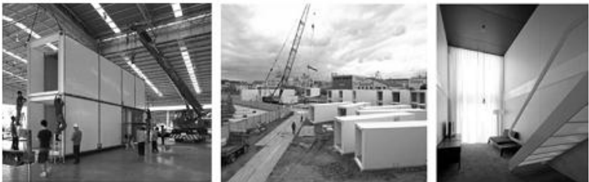
Figure 60 The complete assembling of "Ex-container" in factories (Source: HBRC Journal, 2014)
