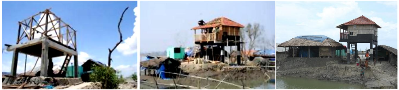
Figure 30. The timber-concrete structure taking shape (Source: Springer, CCA)
