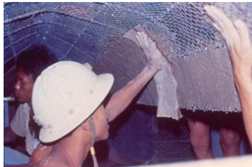
Figure 100. Ferro cement construction process (adpc report, 2005)
