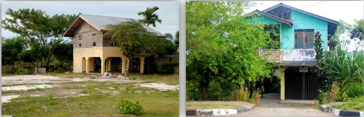
Figure 64. The 2-storey homes with wooden top floors and raised ground floor on RCC columns. The ground floors can be utilized for storage of livelihood items or support small businesses (Source: https://placesjournal.org/ )
