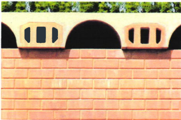
Figure 26: Wall of CSEB
