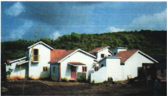
Figure 37: A general view of the housing with the low-lying hills in the background
