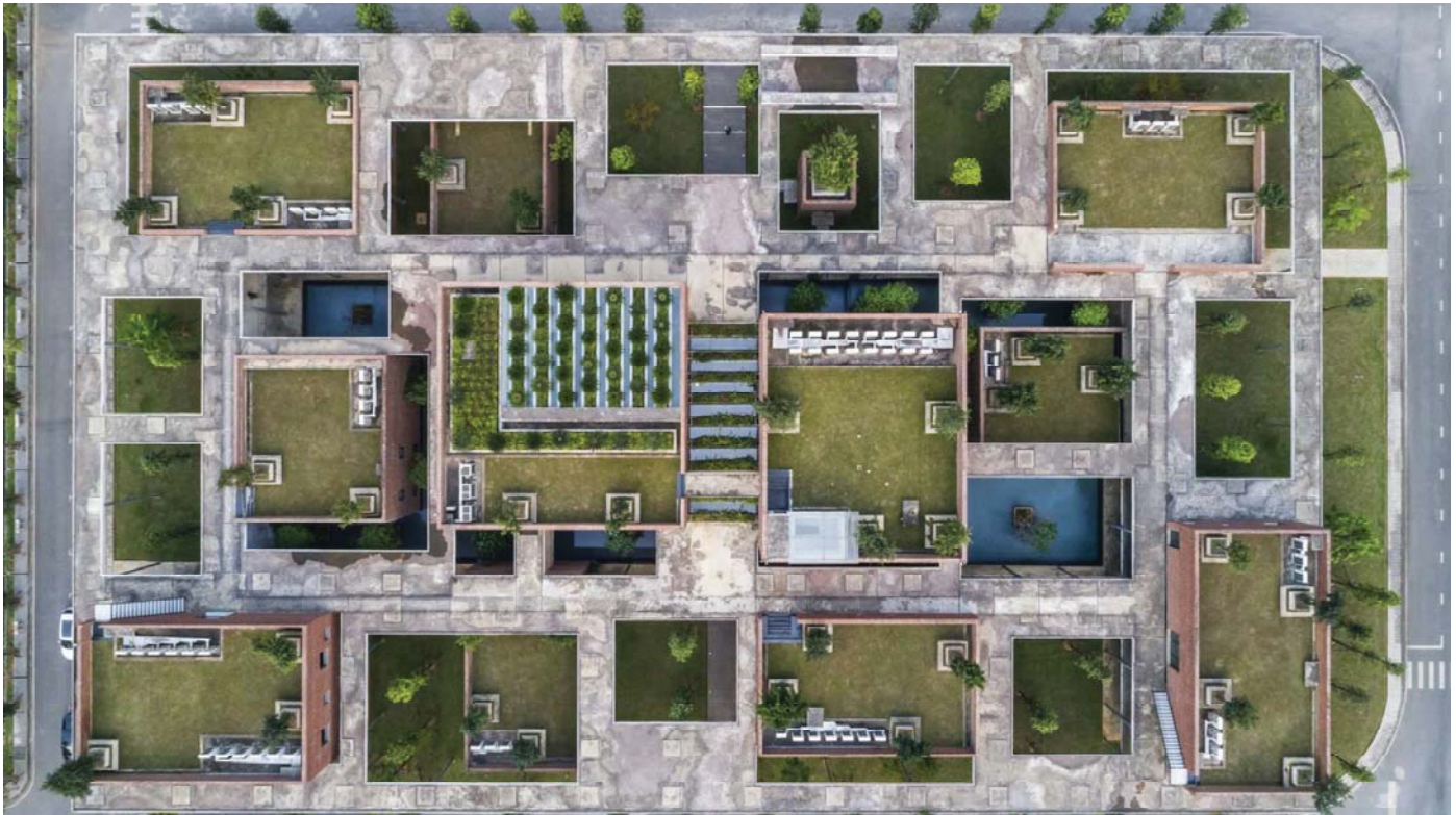
Figure: Photograph of Viettel Academy Educational Center( Source: https://www.archdaily.com/916067/viettel-academy-educational-center-vtn-architects )
