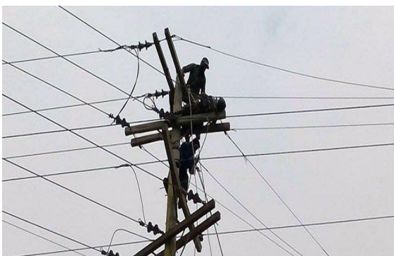
Fig: Electrician at Work
