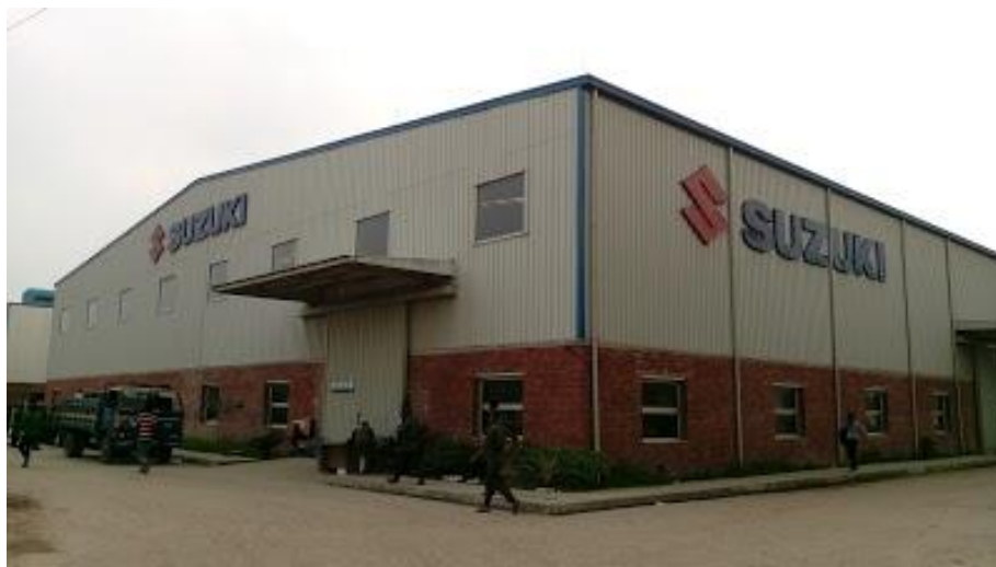
EXHIBIT: RMBL FACTORY IN GAZIPUR
