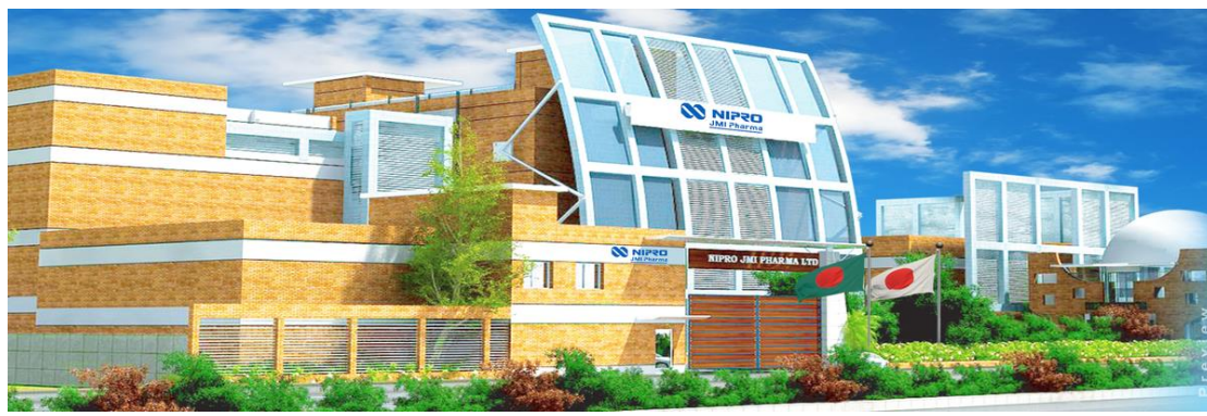
Figure 2 NIPRO JMI Pharma manufacturing plant
