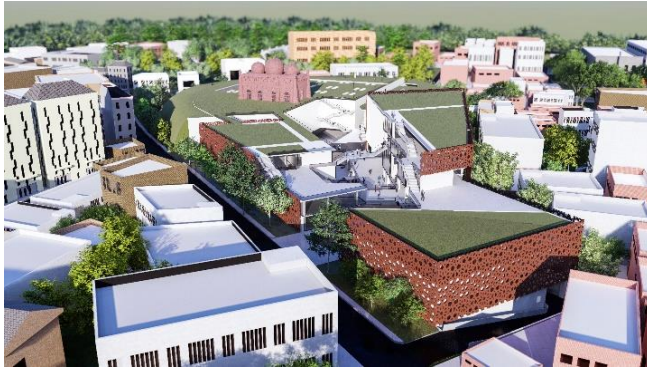
Figure 66 Aerial view of the complex
