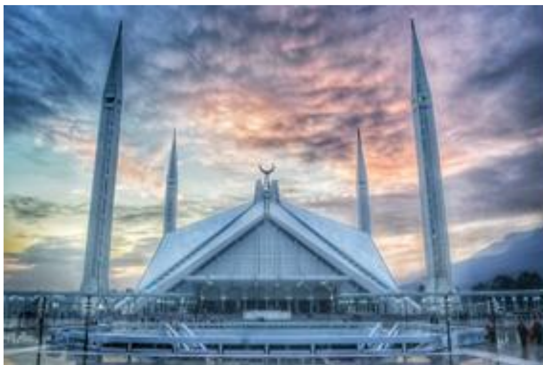
Figure 40 Exterior of the mosque
