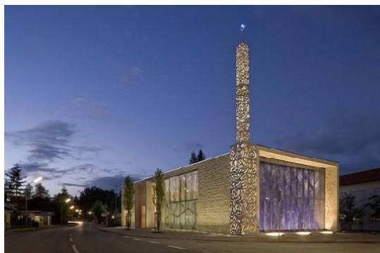
Figure 48 Exterior of the mosque
