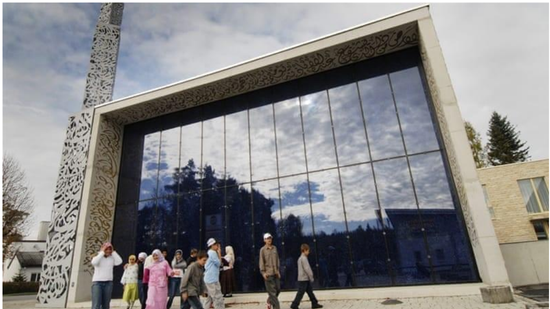
Figure 52 Exterior of the mosque
